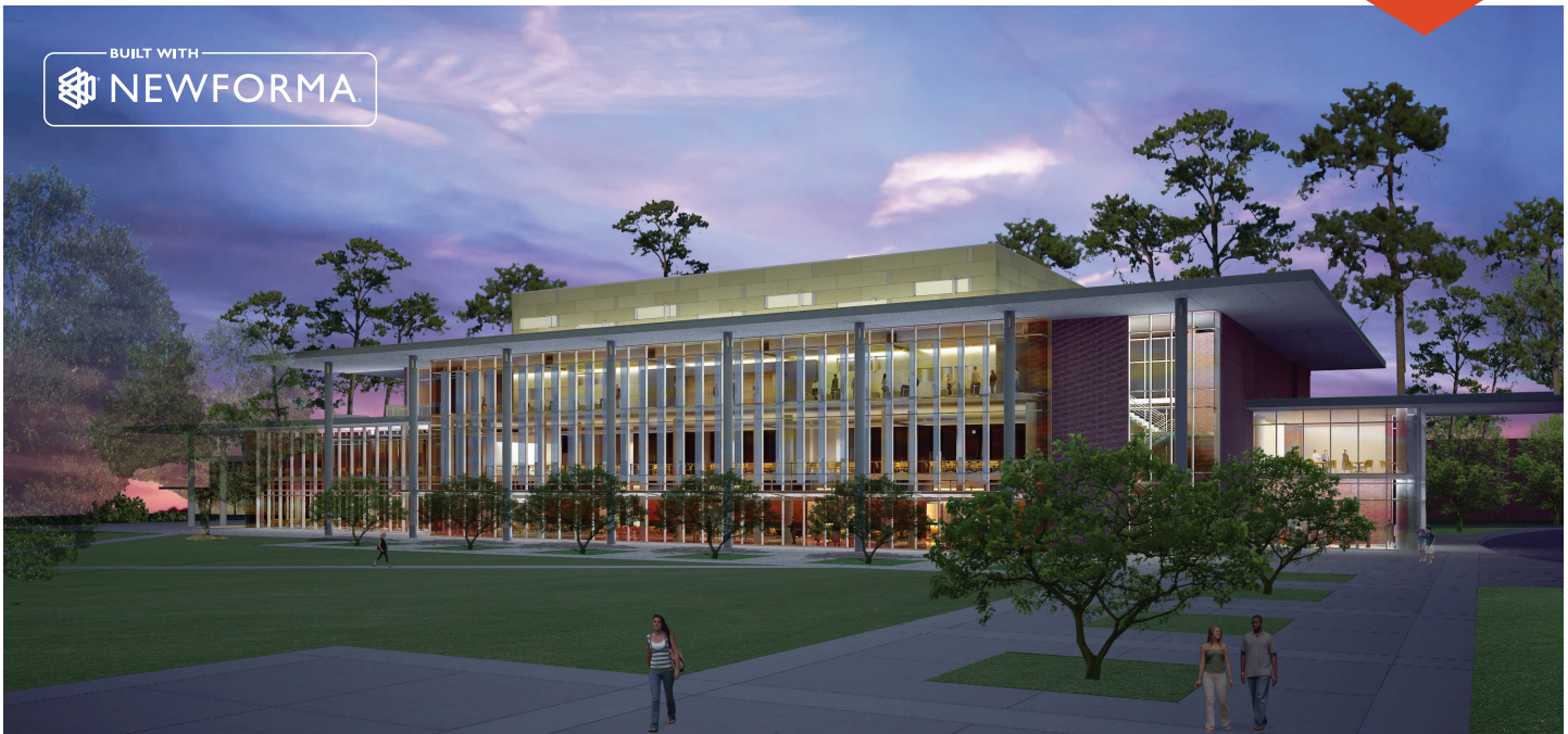
Southeastern Louisiana University Student Union, Hammond, Louisiana, USA
